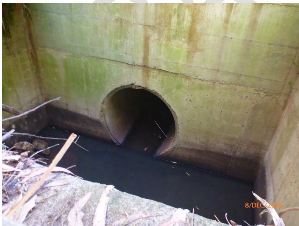
Figure 3-10 Upstream side of 1800mm diameter Yanko Road culvert
