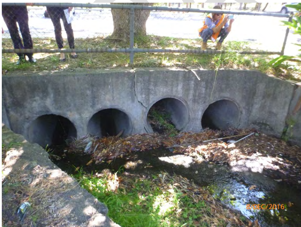
Figure 3-2 Upstream side of 4x 750mm pipe crossing of Lofberg Road
