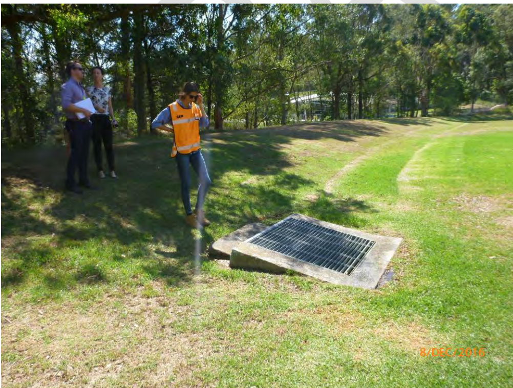
Figure 3-4 Existing downstream basin pit inlet
