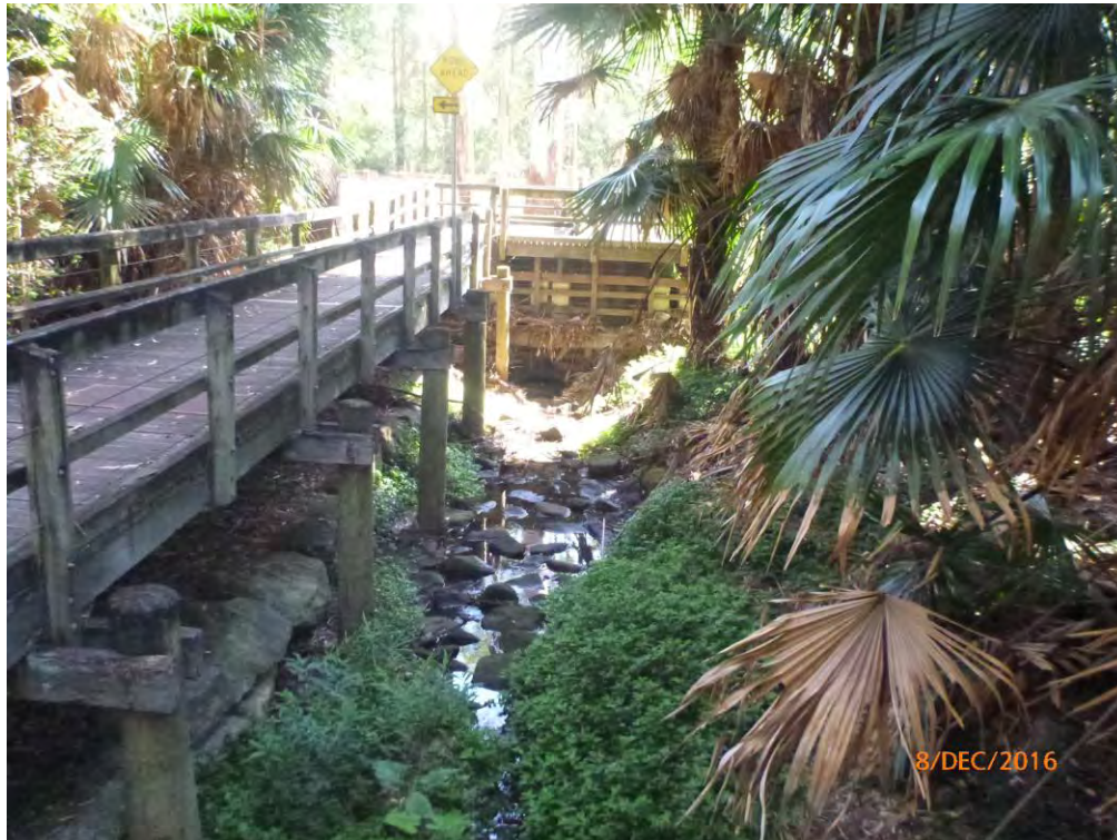
Figure 3-10 Upstream side of 1800mm diameter Yanko Road culvert
