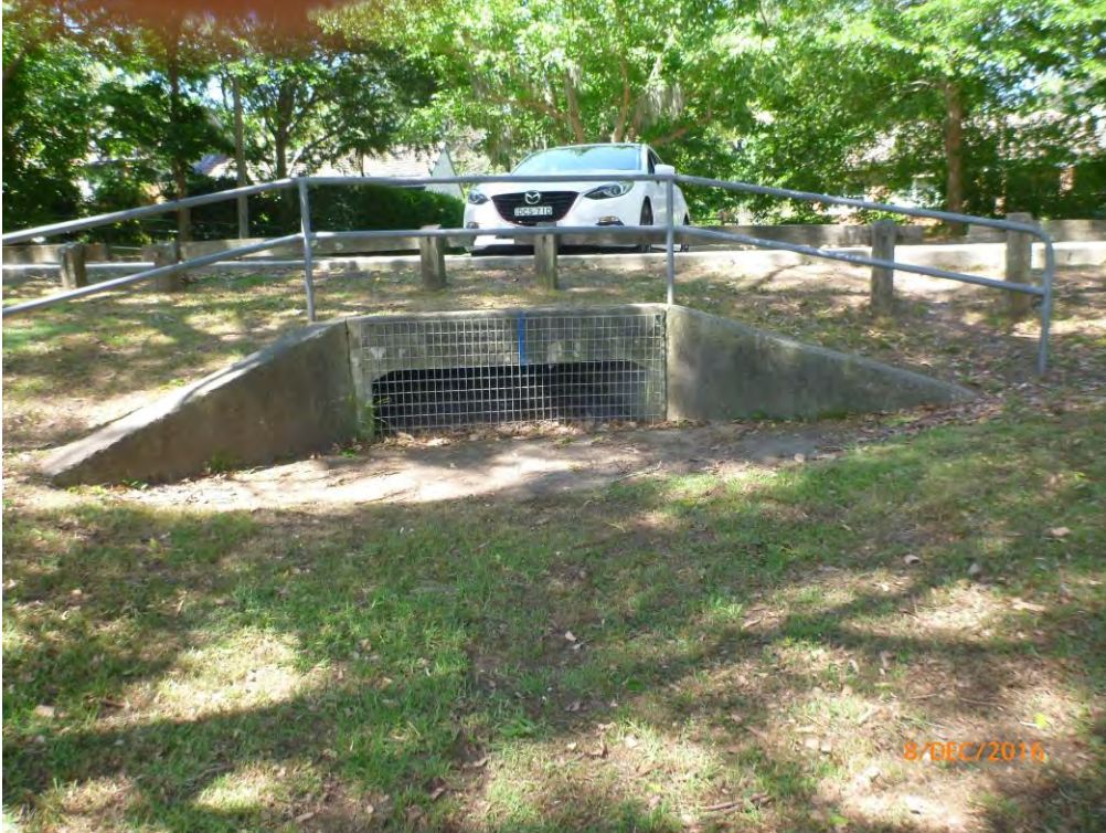
Figure 3-4 Existing downstream basin pit inlet
