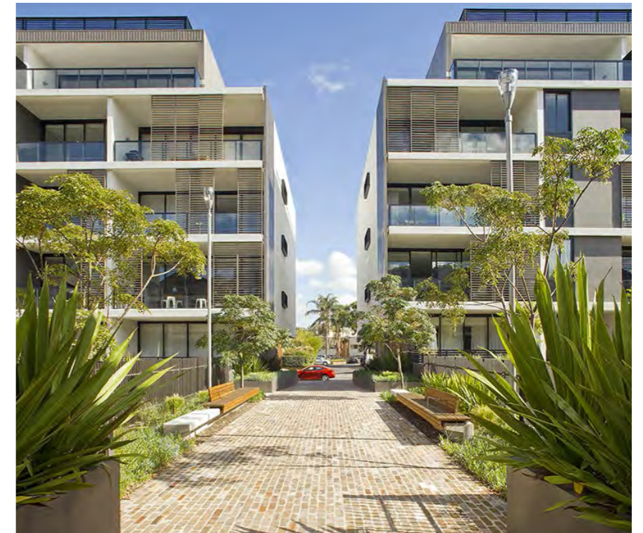
Gantry Apartments, Sydney
