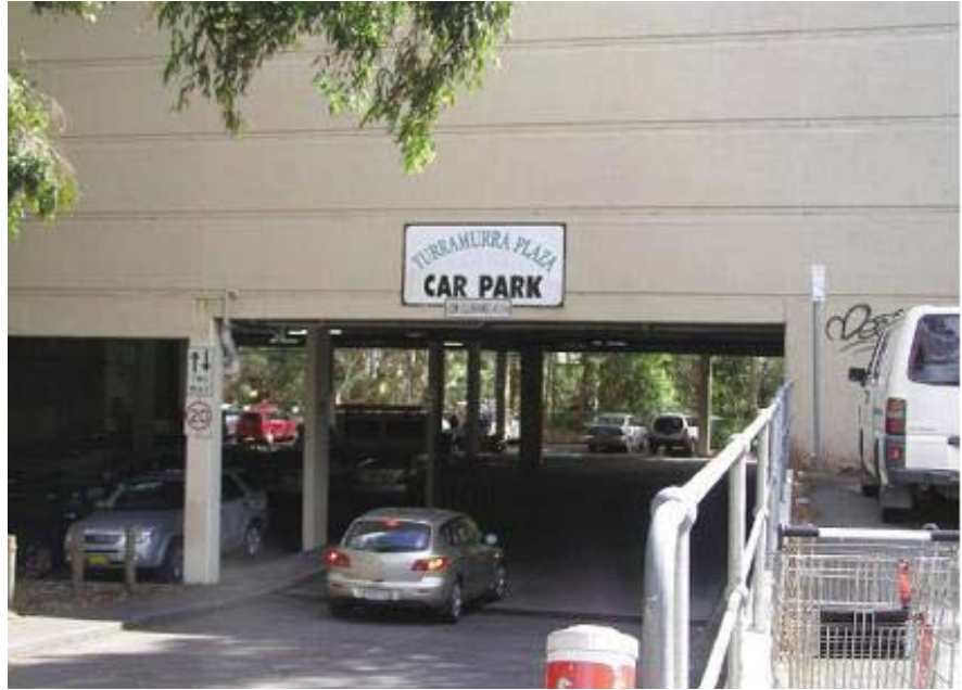
Figure 6.11-1: Turrumurra Plaza Car Park.
