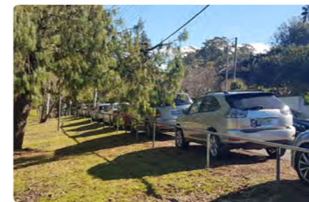
Perimeter barrier rail
