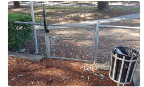
Chain mesh fence
