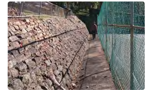
Stone retaining wall
