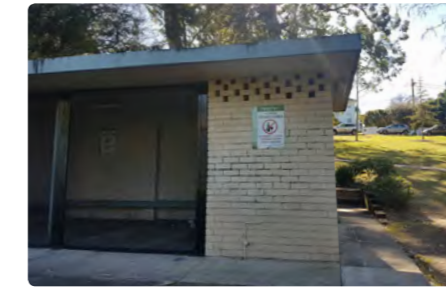
Seating shelter within amenities block with locked screens
