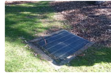
Grated stormwater pit
