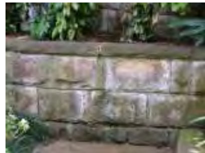
Figure 8 Cracks resulting from minor movement.
