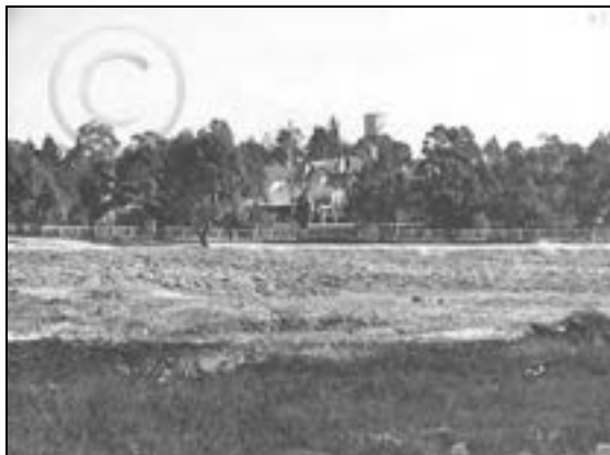
View across Wahroonga Park towards Railway station. Park partly ploughed. June 1927
