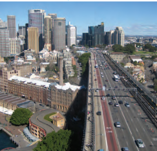
Bradfield Highway on approach to Cahill Expressway
