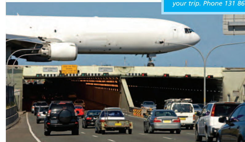
Sydney Airport Tunnel
