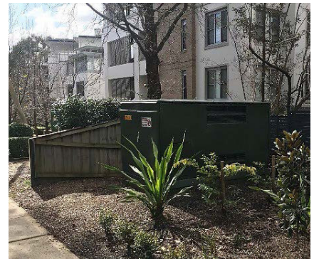
Figure 23.6-4: Kiosk Substation orientated perpendicular to property boundary to minimise visual impact
