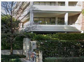
Figure 23.6-3: Hydrant and Booster Assembly located perpendicular to the street to reduce visual impact
