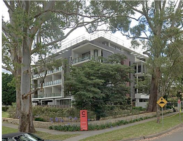
FROM THIS – apartments in Ku-ring-gai
