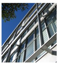
Figure 8C1-2: Retractable shading devices to the windows for solar access control.
