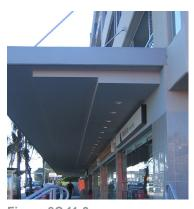
Figure 8C.11-3: Suspended steel box section type awning with under awning lighting.
