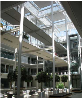
Figure 9C.2-1: Atrium to provide natural ventilation.
