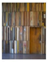
Figure 23.3-1 Recycled timber wall as a feature in the entry lobby.
