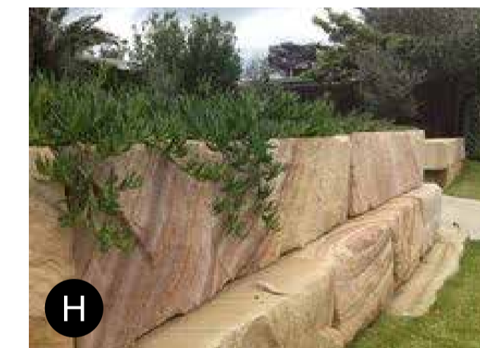
H Sandstone terrace retaining wall
